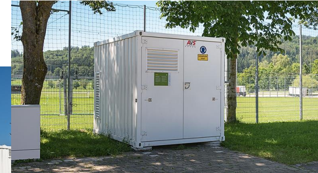
Diesel generator 90kVA
