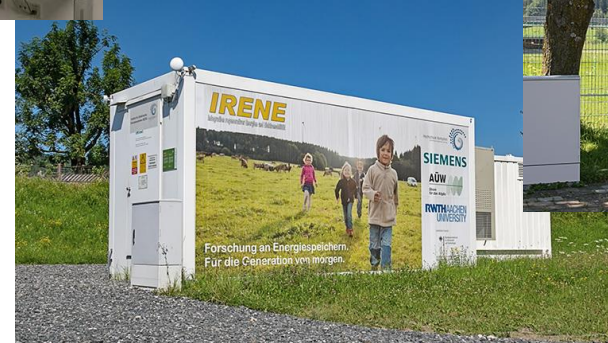
Battery storage 240kVA
