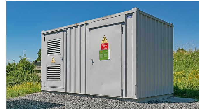
Transformer station IRENE
